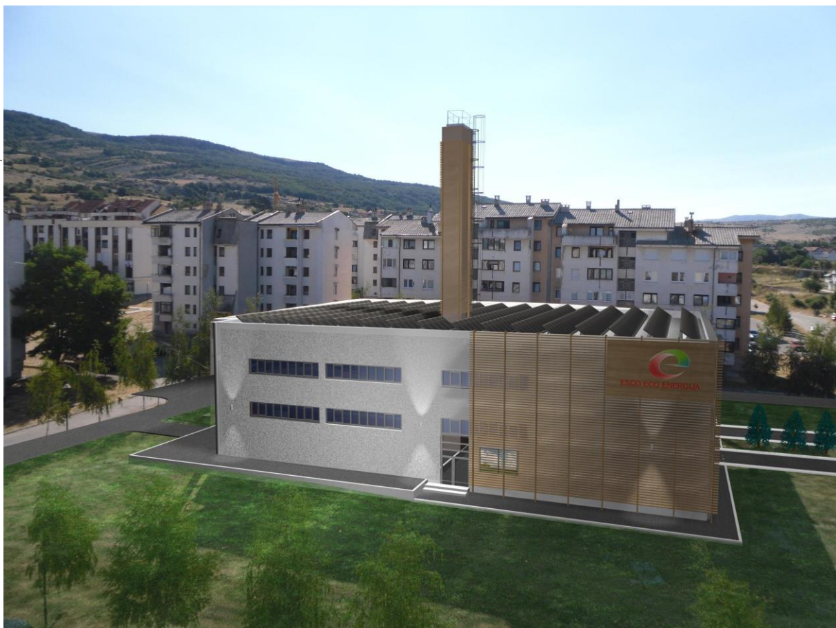
ENERGY PARK LIVNO, BOSNIA AND HERZEGOVINA, CHP 1,4MWel , PV 100kW...
